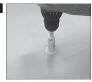
Make a 3/4" hole in vehicle where center of antenna will be located.
