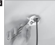
Tighten nut two turns after contact to inside surface.
