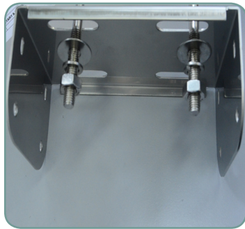
Position of the U-bolts, nuts and washers
